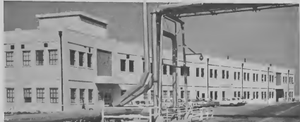
EAST WING, top and ground floors of the Lab, contain the Analytical/Development Section. The Inspection Section is on the west end (left).
